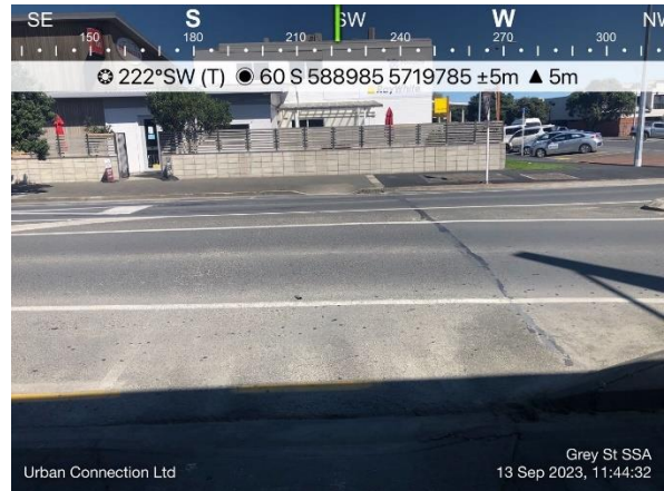
Figure 5.3-13 – Missing tactile pavers at crossing points across Childers Rd (east of Grey St)
