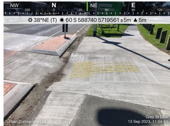
Figure 5.3-8 – Directional tactile not covering the whole footpath width
