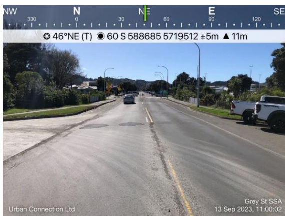
Figure 5.3-9 – Missing advance warning diamond symbol marking
