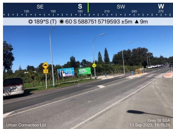
Figure 5.3-10 – Missing reflectorised orange disc
