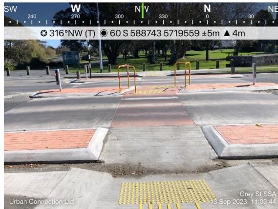
Figure 5.3-7 – Narrow crossing and refuge, long ramps and faded zebra markings
