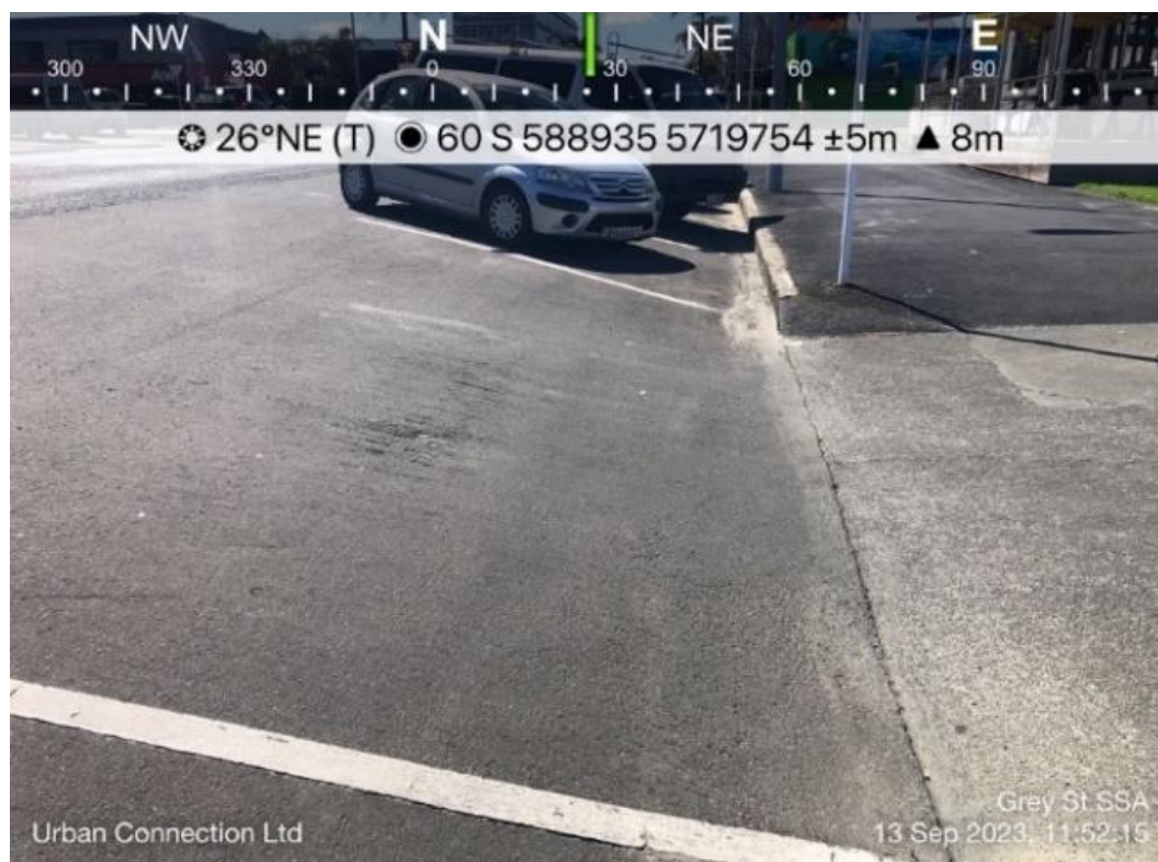
Figure 5.3-5 – Steep crossfall along Grey Street
